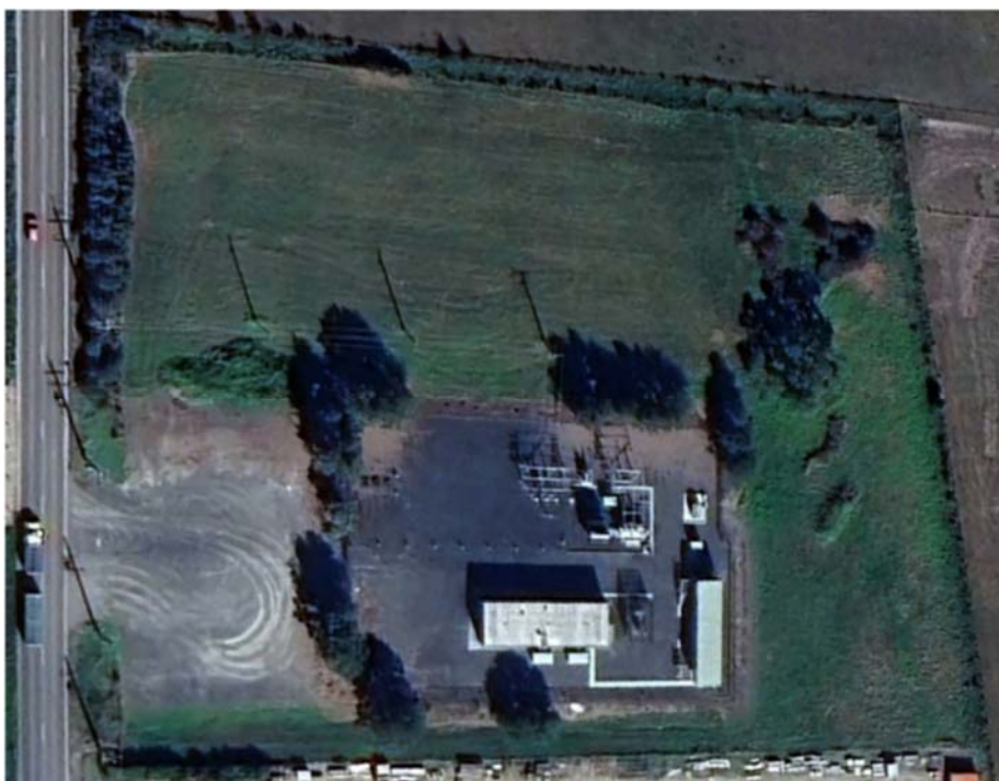
Figure 13 : Lang Lang zone substation site
