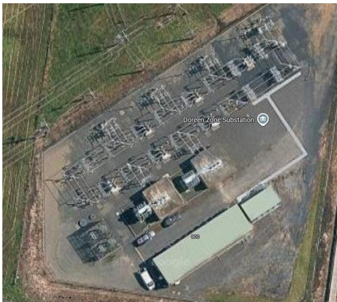
Figure 5: Existing Doreen (DRN) zone substation site
